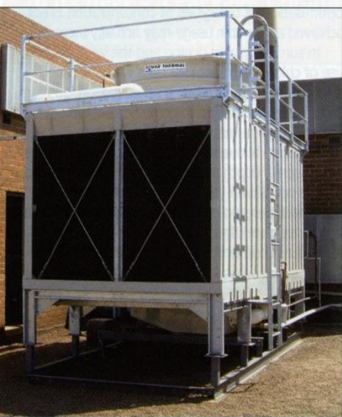
Crossflow cooling tower
